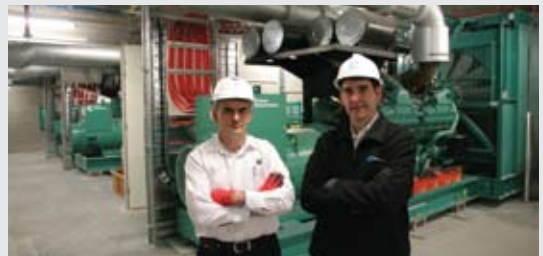
Adam Ferrara, Contracts Manager for the Cummins Power Generation team in Melbourne (left) with Nathan Saffery, Project Manager of PSG Elecraft.
